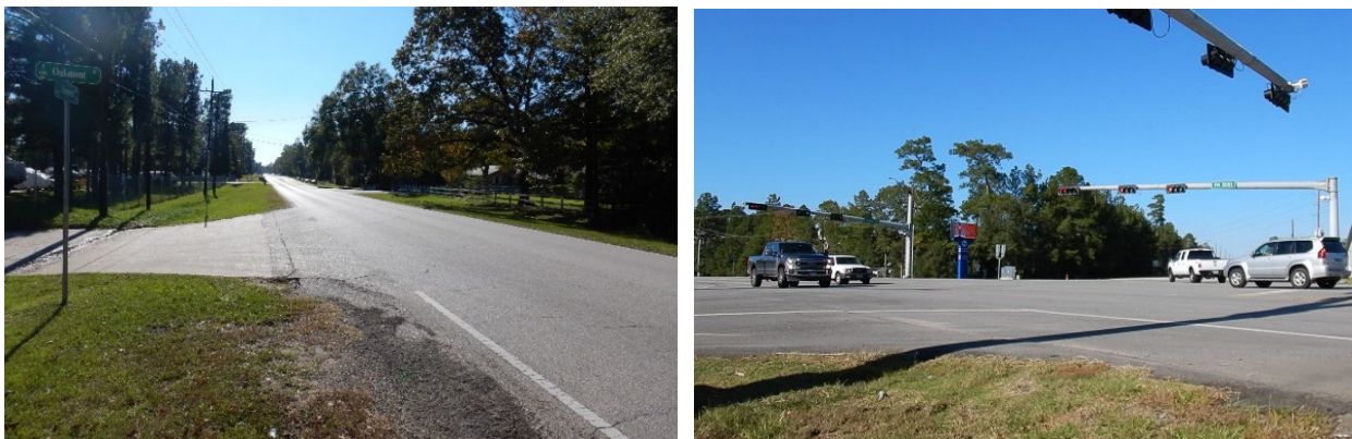
Figure 15 Typical intersection on Airport Rd with no crosswalks
