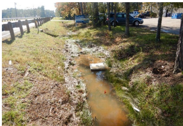
Figure 14 Water retention in ditches
