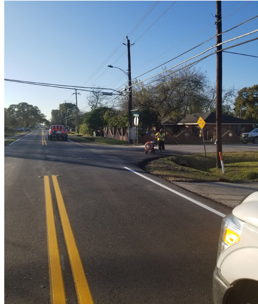
Completed Street Rehab
