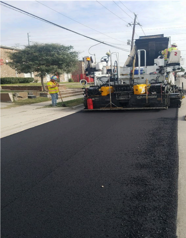
Placing New Surface
