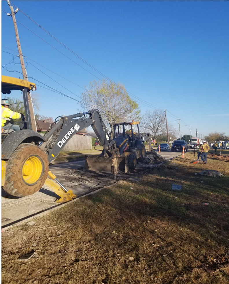
Remove Sections of Base that Need Replacement
